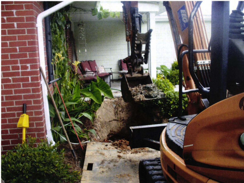
Picture 2: UST 346Ash excavation in progress.
